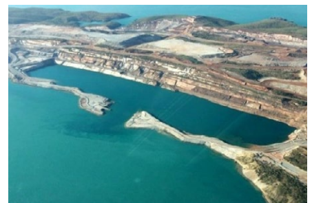
Above: Bingham Canyon Manefay Slide. Complete destruction of the highwall, haul road and part of the heavy vehicle workshop.
