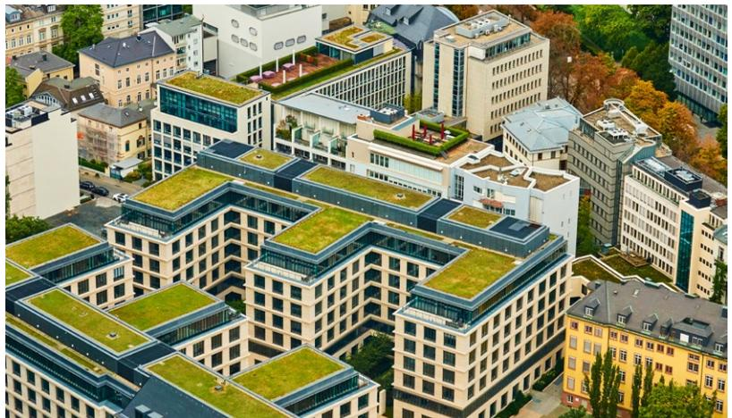
points included. The impact of roof gradient on the density of growth media and its propensity to shift or slide should be considered for heavy rain events.
